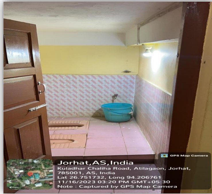
A hygienic attached toilet in Girls' Common Room
