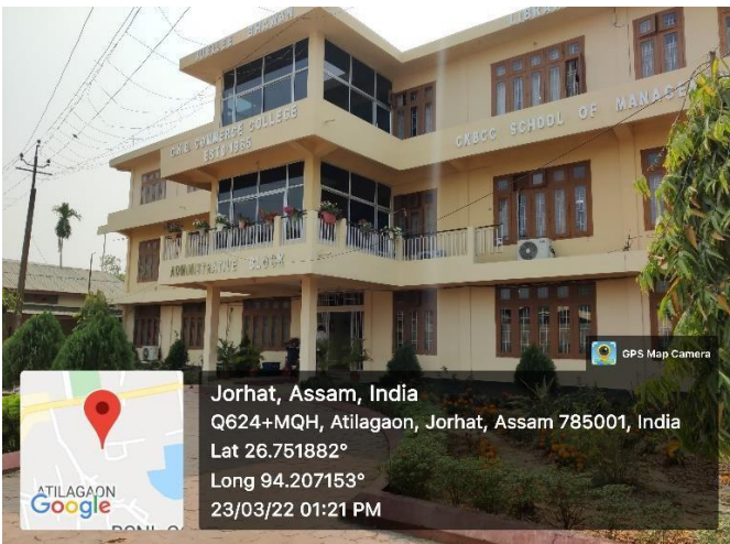
COLLEGE ADMINISTRATIVE BUILDING
